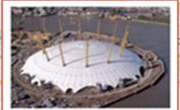
NORTH GREENWICH ARENA (The O2)
